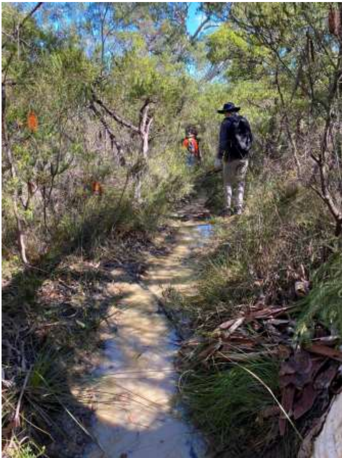
Drainage work on the Mooray track Heathcote NP
