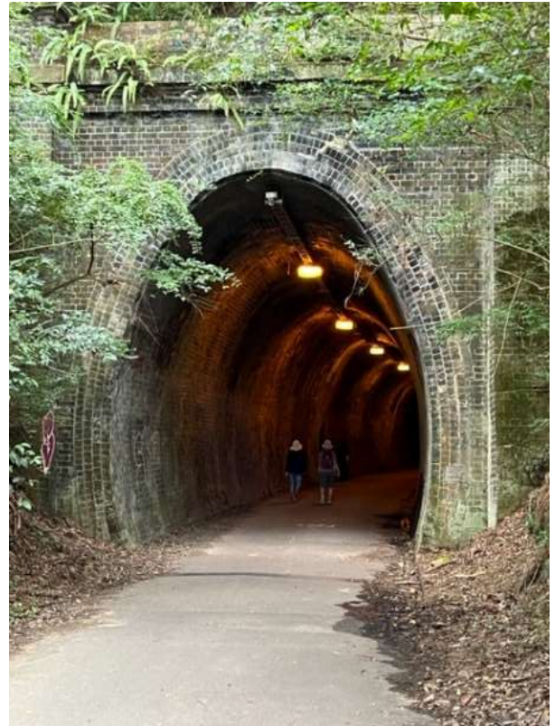
Fernleigh rail tunnel
