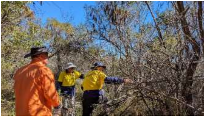
Trimming the scrub over the track
